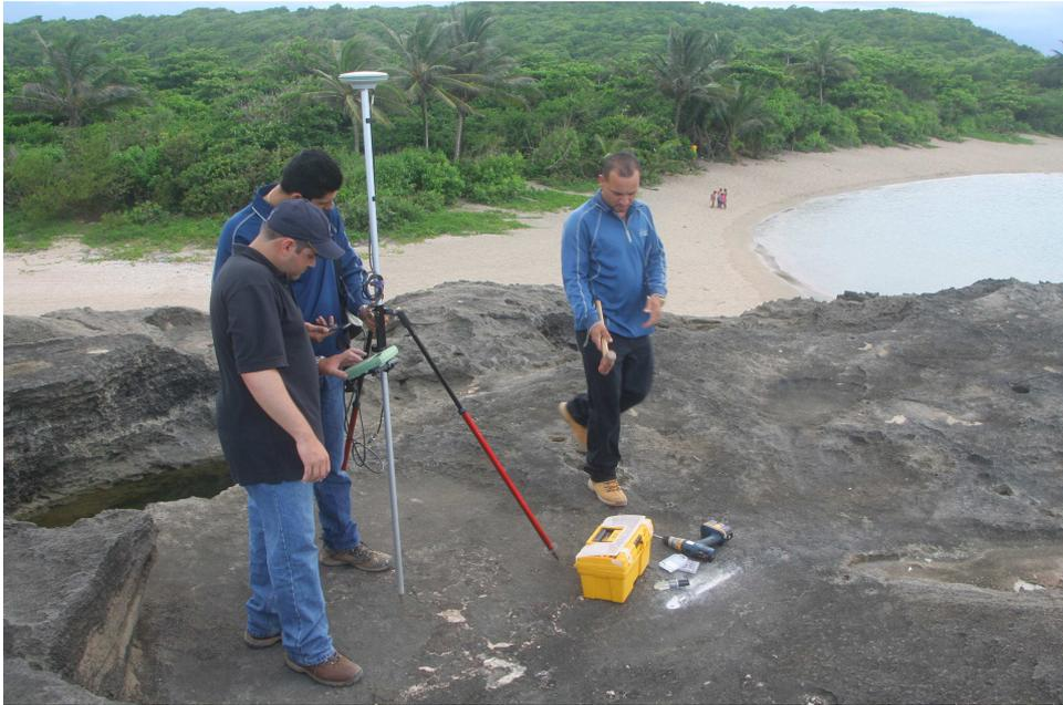
Figure 31: Employees of Vernix Engineering installing and measuring Punta Manatí benchmark.
